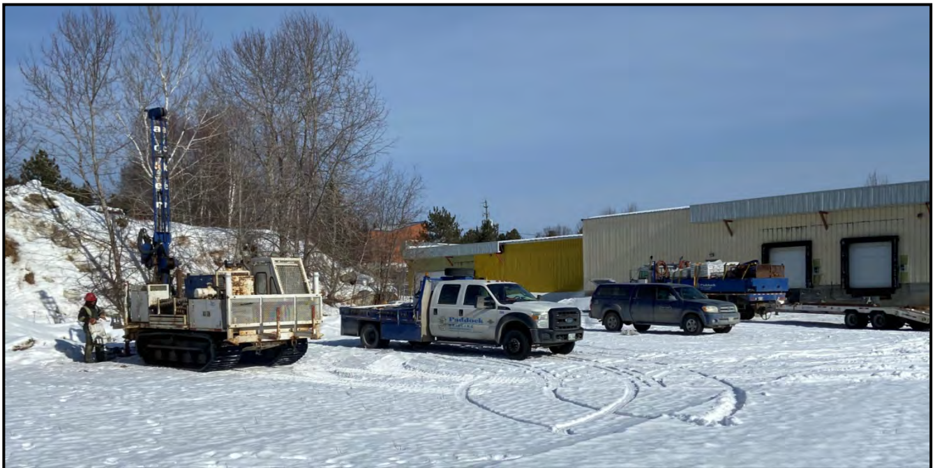
PHOTOGRAPH #2: Drilling TH2 as seen facing north-northeast.
