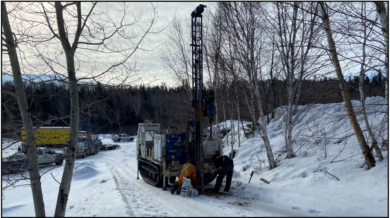
PHOTOGRAPH #1: Drilling TH1 as seen facing south.
